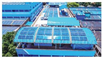
Laboratory & Allied, 1.2 MWp grid-tied solar plant
