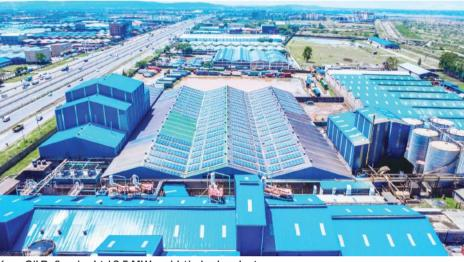
Kapa Oil Refineries Ltd 2.5 MWp grid-tied solar plant.
